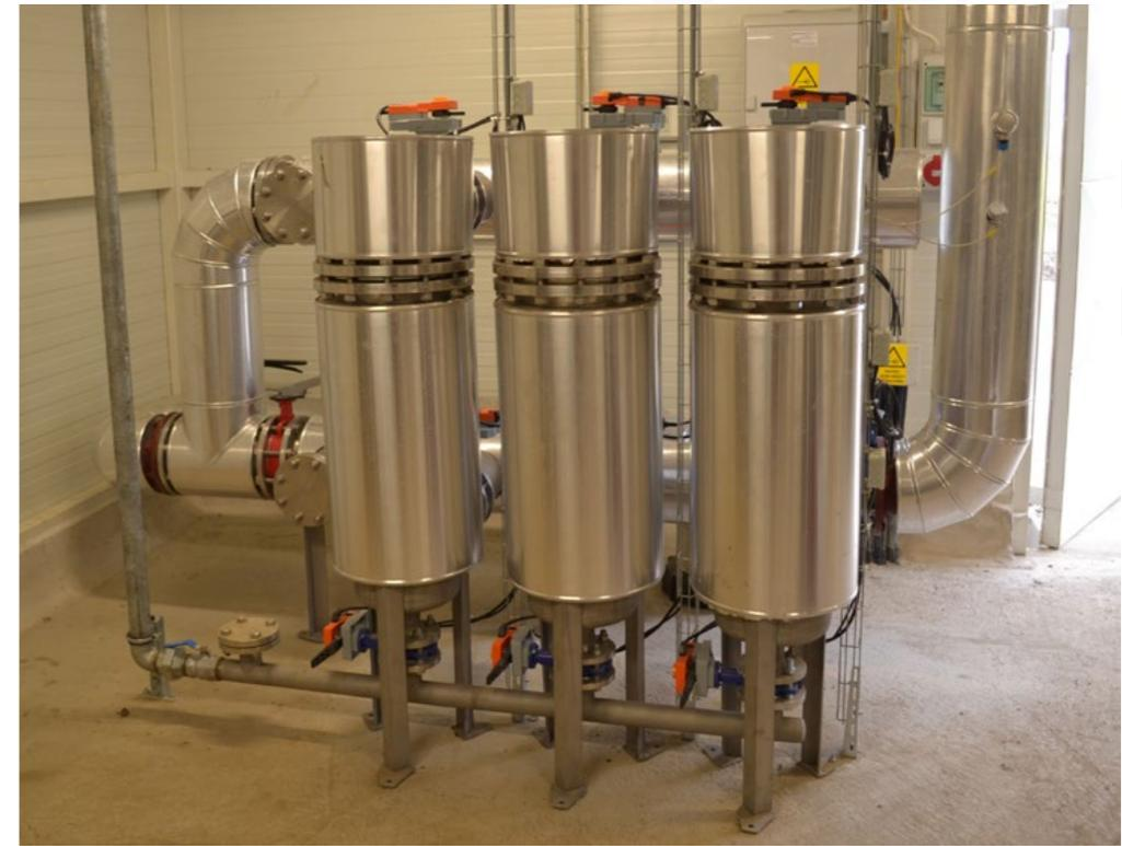
The iron filters for reinjection
