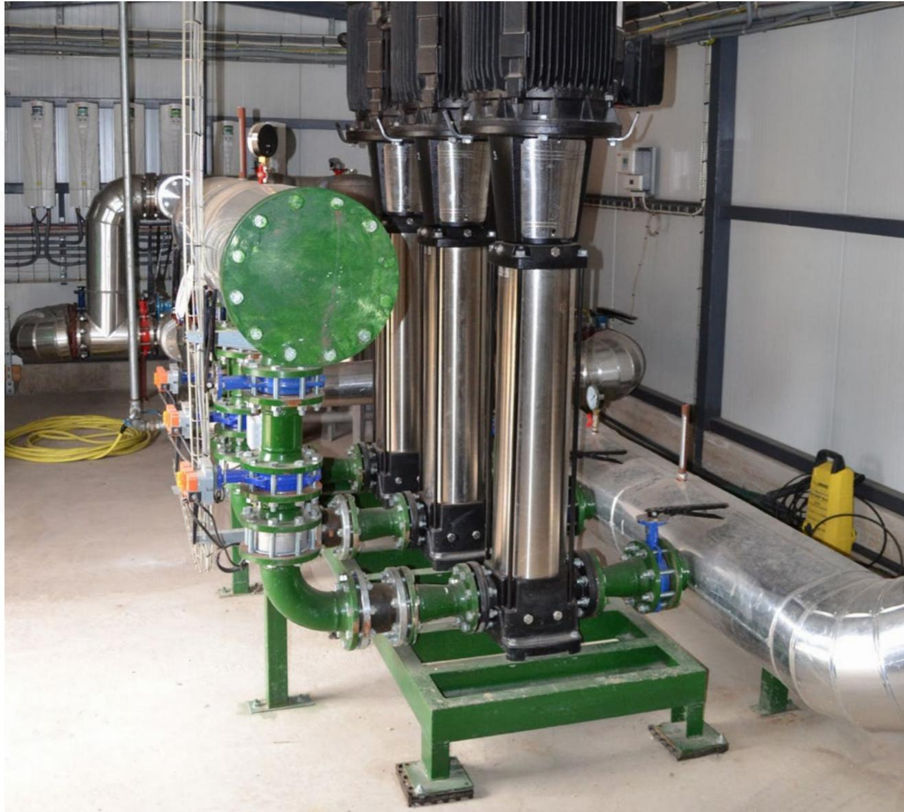
*Pump station for reinjection wells*
