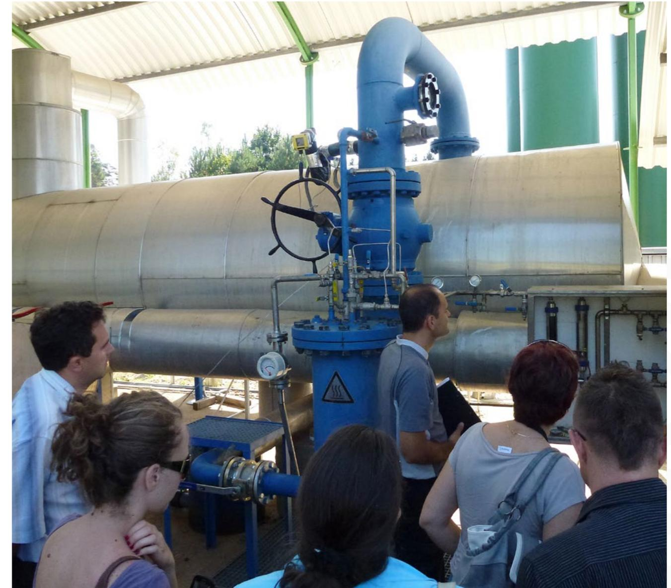
*Production well of a doublet in a carbonate reservoir in Bad Blumau, Austria, with a degassing unit*
